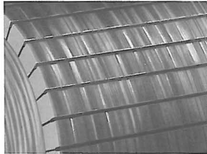
STREAKING on the commutator surface signals the beginning of serious metal transfer to the carbon brush. Check the chart below for possible causes.
